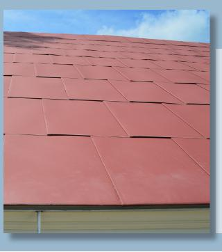
Stainless steel has a major advantage in that it is more efficient at reflecting solar energy than typical roofing materials. These include painted surfaces, rubber and plastic membranes and bare metals like aluminum, copper and zinc develop oxides or patinas that convert solar energy to infrared wavelengths.
