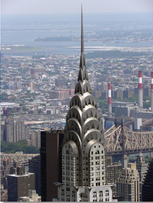
The best performance of all comes from the use of hydrophobic stainless steel surfaces that resist the accumulation of dirt, maximizing solar reflectance and minimizing the need to clean the roof or façade. Accumulated surface soil absorbs more solar radiation than it reflects. It is, therefore, important to keep the stainless steel clean in order to maintain maximum solar reflection. The use of a hydrophobic surface will delay, if not eliminate, the need to clean the building's surface.
